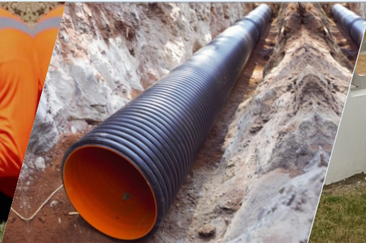
Underground Sewer Pipe Line
