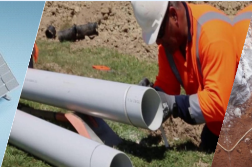
Underground Water Supply Pipe Line
