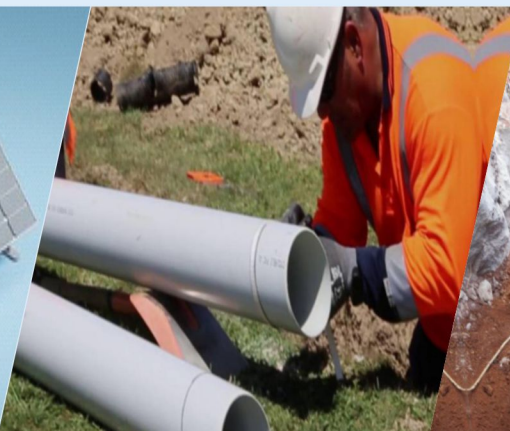
Underground Water Supply Pipe Line
